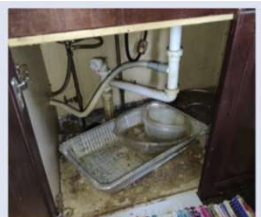
Leaky Plumbing Replaced - Before
