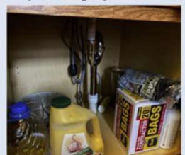
Leaky Plumbing Replaced - After
